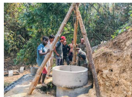
Installing the tubewell
