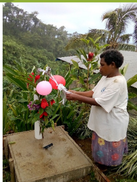
Preparing the slab for the water tank at Torlie Kindergarten, Pentecost.
